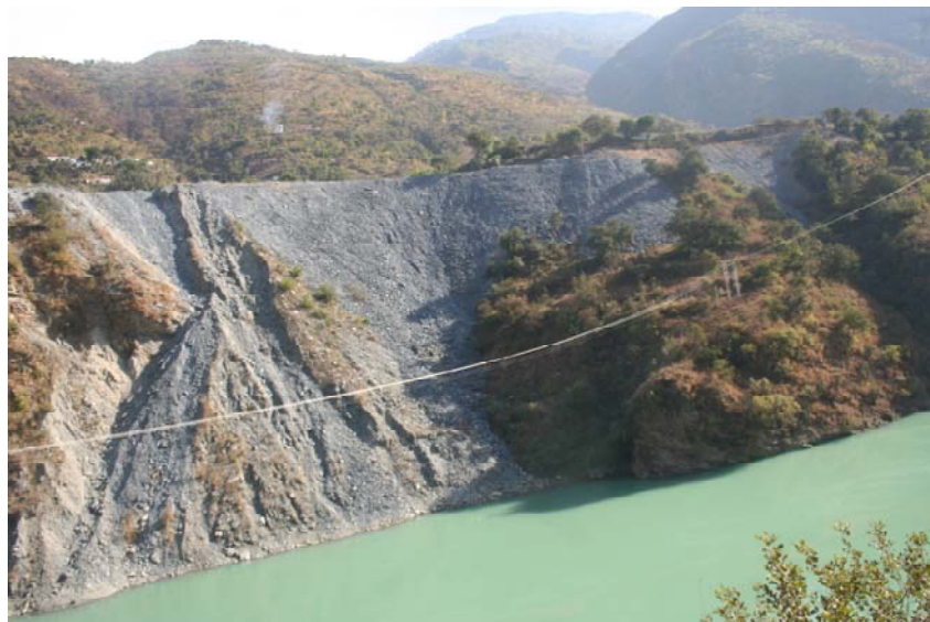
Fig. 2.4b Muck dump site downstream of Tehri dam along the left bank of Bhagirathi river
