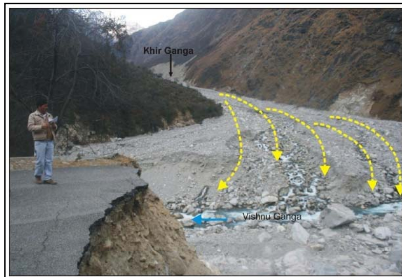
Fig 17: Debris flows at the confluence of Khir Ganga with Vishnu Ganga near Hanuman Chatti. Vishnuprayag project is located ~1 km downstream from this location
