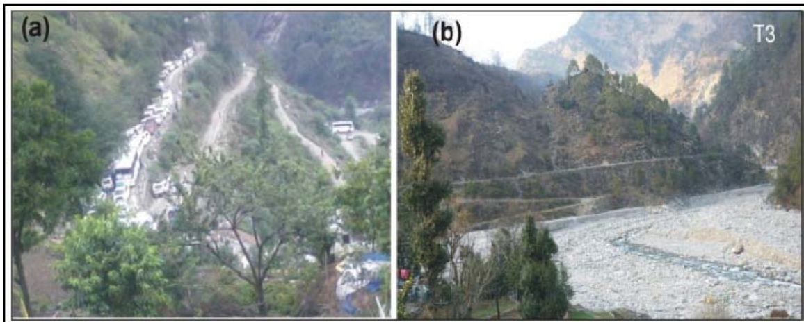
Fig. 3.14: The sediment spilled over from Sonprayag was trapped at Sitapur which served as a vehicle parking space (for Kedarnath yatris) on the bank of Mandakini river (a). Note the magnitude of valley-fill aggradation (b). Note the hairpin bends of the road with vehicles before the flood (a) and without vehicles after the flood (b) gives an idea of the amount of debris being aggraded at Sitapur.
