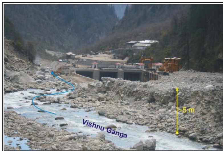
Fig 18: Hyperconcentrated sediment laden water was obstructed by the Vishnuprayag barrage which caused a temporary lake. The lake finally breached along the weak debris laden left flank. As a result the sudden sediment laden flood surge caused large-scale damage downstream (Pandukeshwar and Govindghat).
