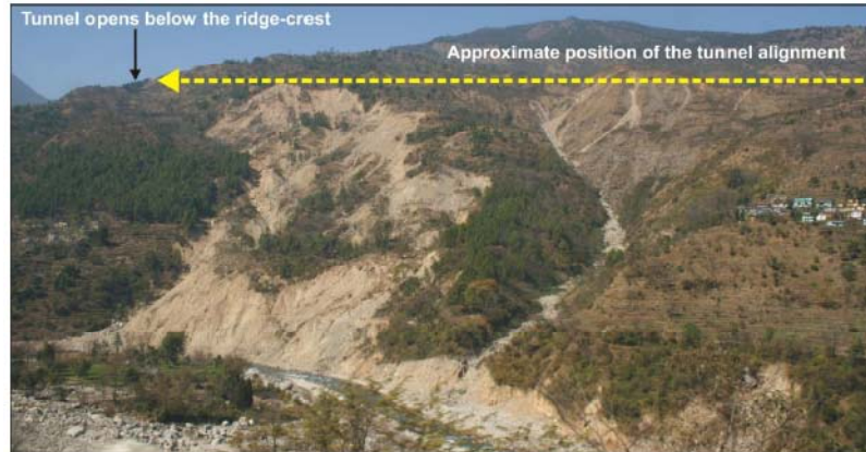
Fig. 2.9: Landslide located on the NE-SW trending ridge along the Mandakini valley. The head race tunnel opens behind the crest of the ridge (along a seasonal stream which is also the muck disposal site of L&T).
