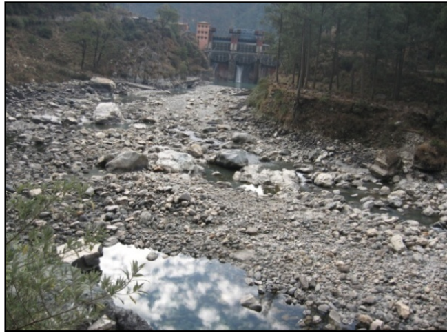
Fig. 2.2a: R. Bhagirathi downstream of the Maneri-Bhali I dam
