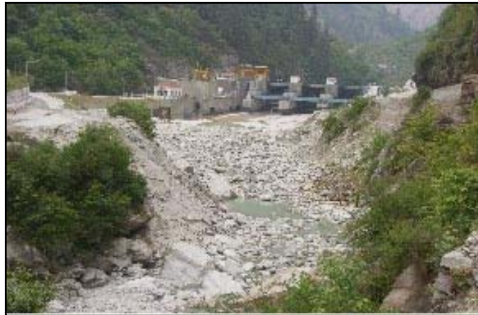
Fig. 2.1: R. Alaknanda downstream of the Vishnuprayag dam in Chamoli district
